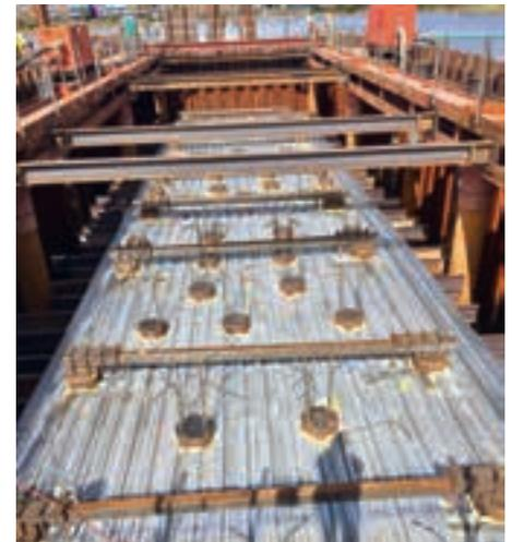
Preparation of concrete slab within cofferdam
