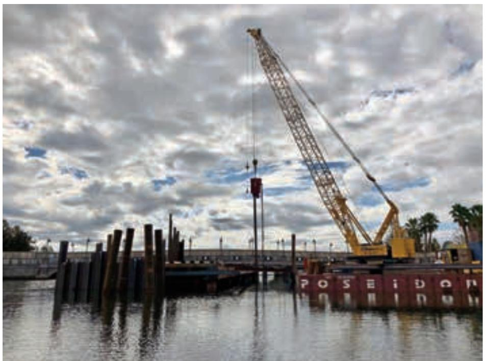
Installation of pipe piles on Hourglass Lake
