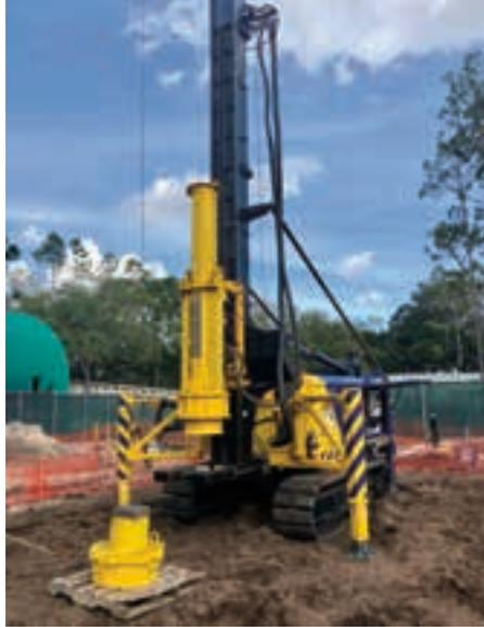
CD-29 rig used to install the H-piles
