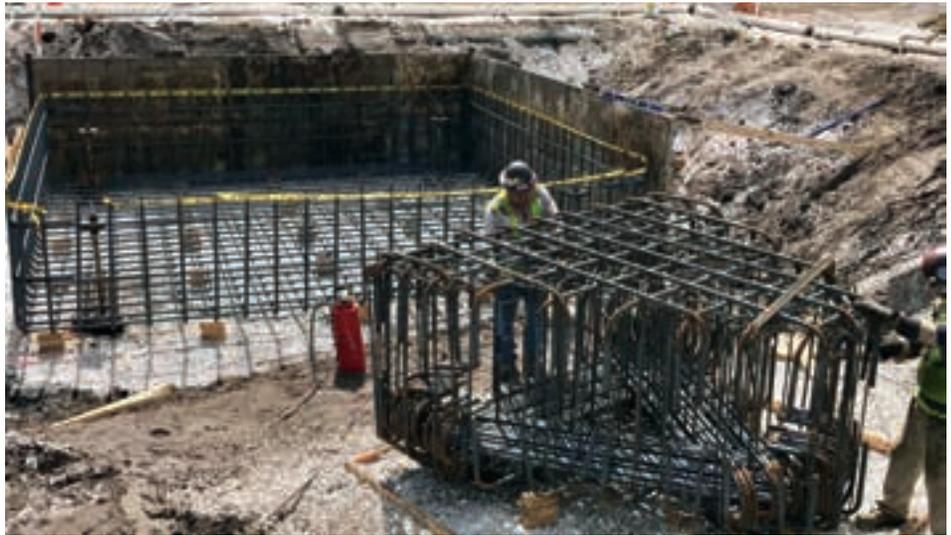
Preparation for construction of a pile cap
